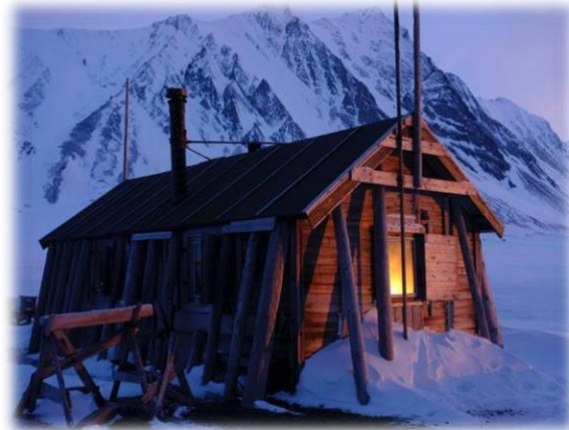
Bamsebu- 20 m 2 Vertical logs were set up to try to prevent polar bears from getting into the cabin.
